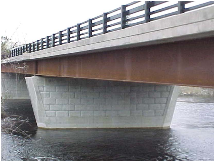
West Bridge, Fairfield-Benton
